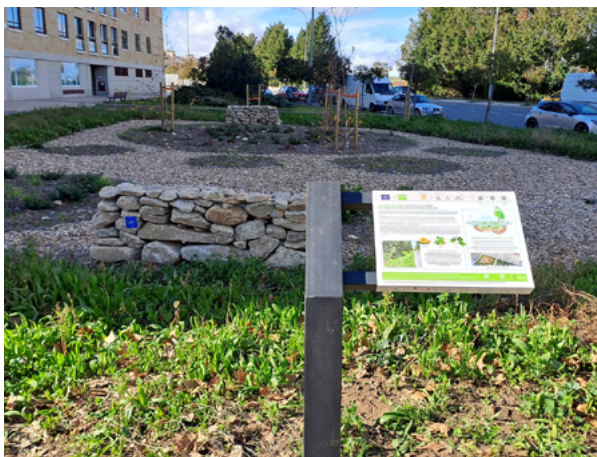
Rain garden and awareness-raising signage in Moreruela street.
