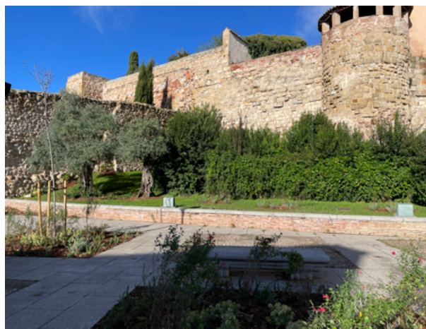
Urban drainage systems and planting in Niños del Coro in heritage area.
